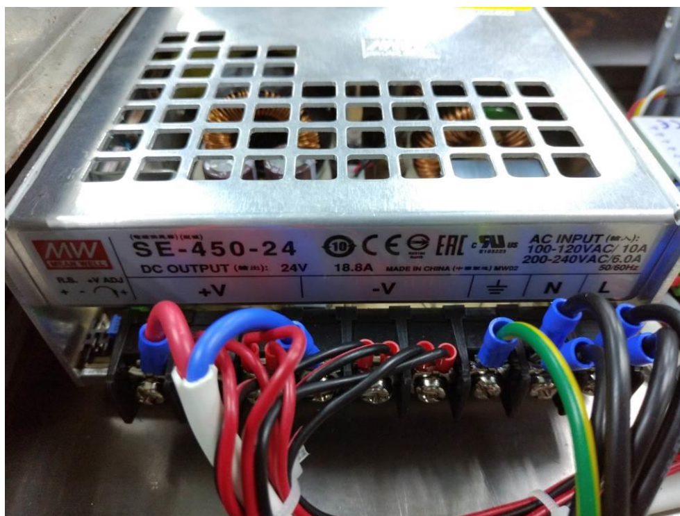
Photo 9: Power Switch view
