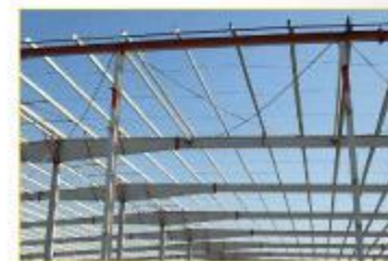
更大的檩条间距 larger purlines distance
