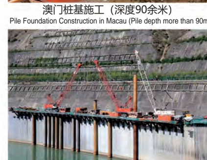
水电站大坝防护桩 Hydroelectric dam fender pile
