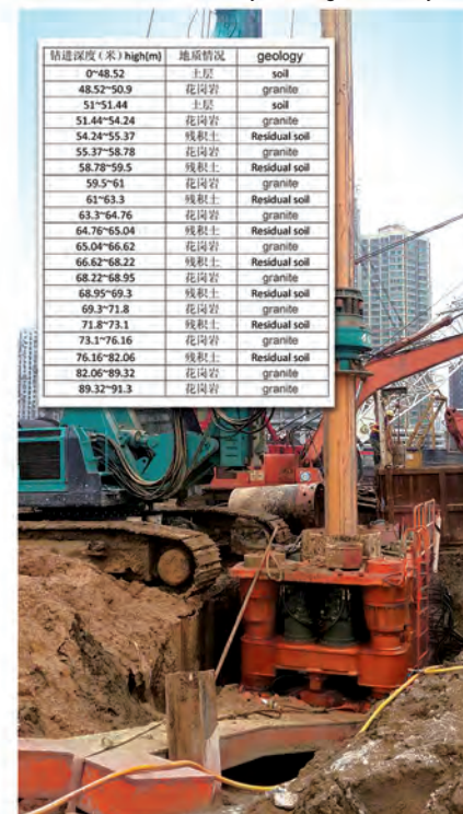
澳门桩基施工 (深度90余米) Pile Foundation Construction in Macau (Pile depth more than 90m)
