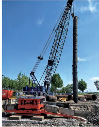
直径1.2米旧桩拔除 1.2 meter diameter old pile remove working
