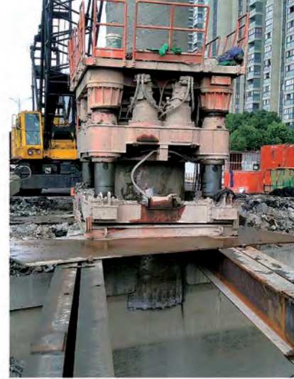
切割钢筋混凝土 Cutting reinforced concrete
