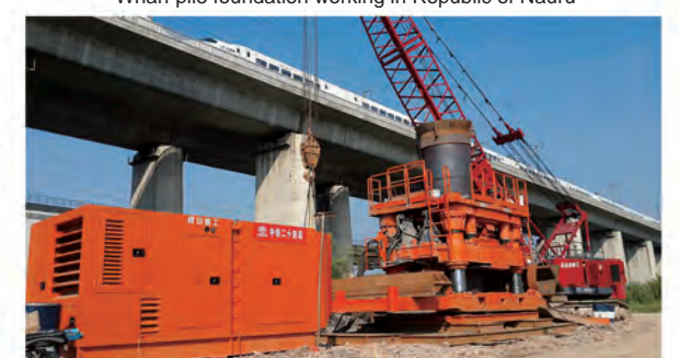
紧邻高铁桥墩施工 Adjacent High-speed Rail Bridge Piers Construction
