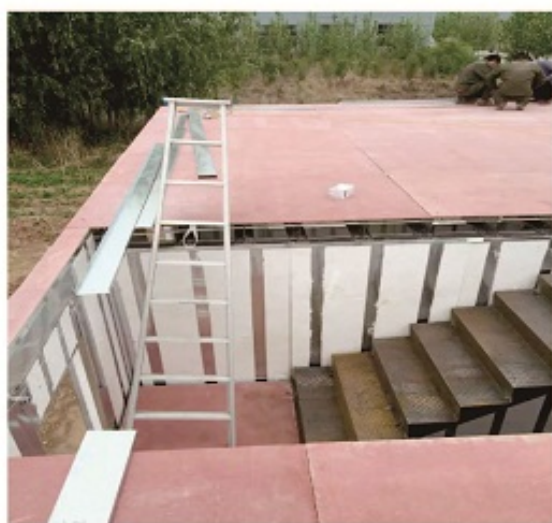
Reinforced MgO board as floor panel
