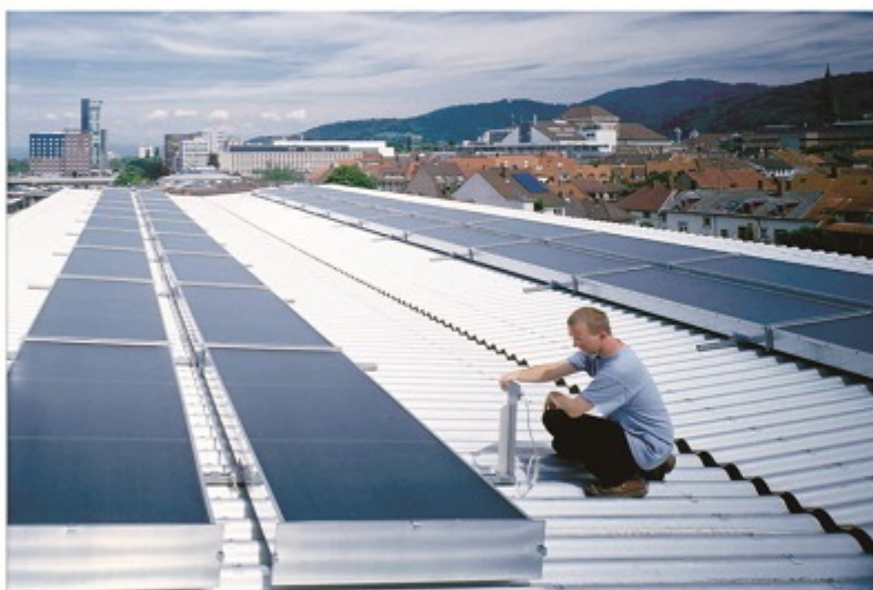
Solar panel on the Aluminium foil MgO roofing sheets
