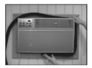
10. Assemble the trim frame by inserting the top and bottom pieces into the side pieces and snapping into place. Slide over the unit face until flush with the wall
